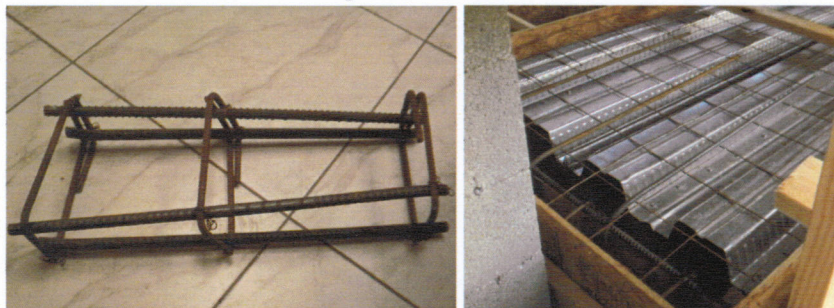
Rebar End Assembly and Rebar End Assembly Installed into Form
