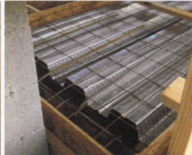
Rebar End Assembly and Rebar End Assembly Installed into Form
